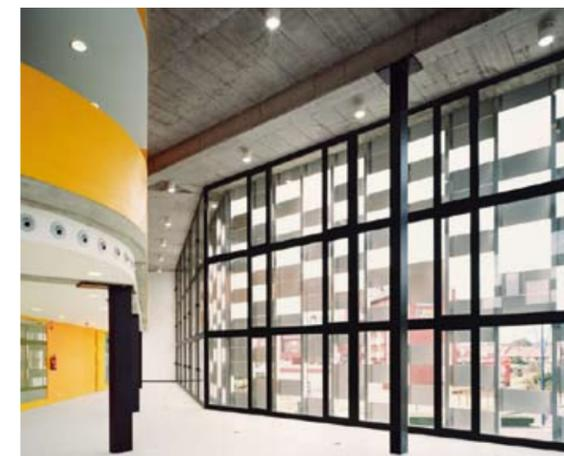
• Inside, the different functions converge towards a single open space without however mixing the routes. On the outside the ceramic skin conjugates the theme of permeable continuity while making it possible to mix the opaque areas with the large glazed surfaces without undermining the building's material consistency or its geometry.
